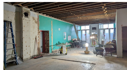
1011 Garfield St lobby under construction
